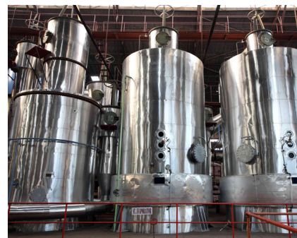
Installations in communicating vessels.
