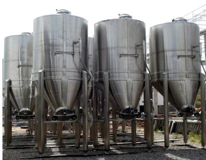
Installations in communicating vessels.
