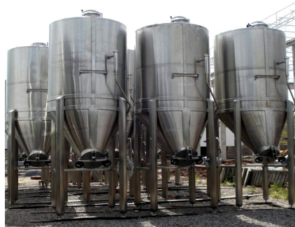
Installations in communicating vessels.
